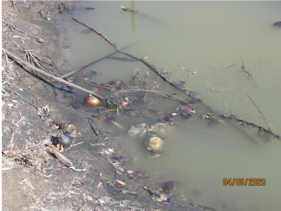
Photograph 71 :Close-up view of Swale #4, note onions and debris.
