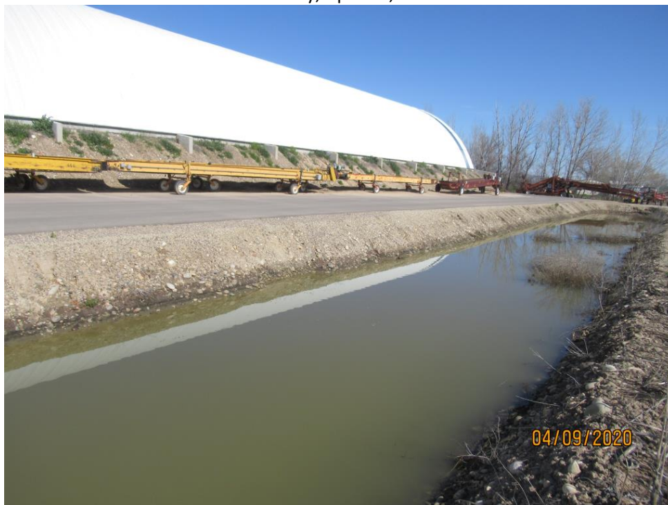
Photograph 31 :Swale #2, mid-way, looking north, note rills along west bank
