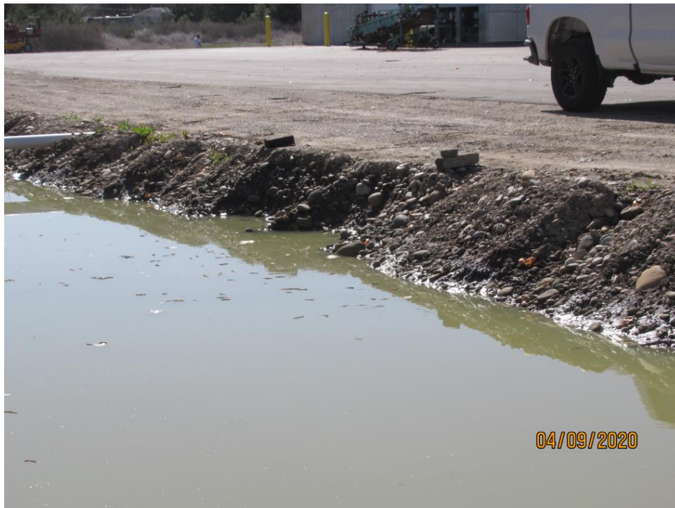
Photograph 56 :Rills on south bank of Swale #3.
