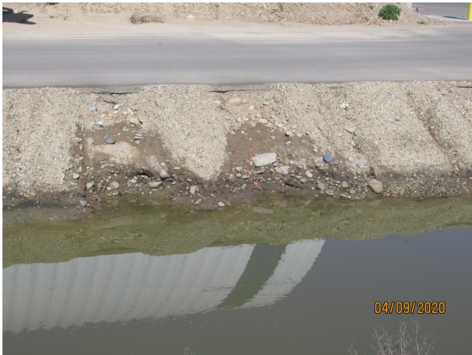
Photograph 34 :Close-up view of north end rills, Swale #2.
