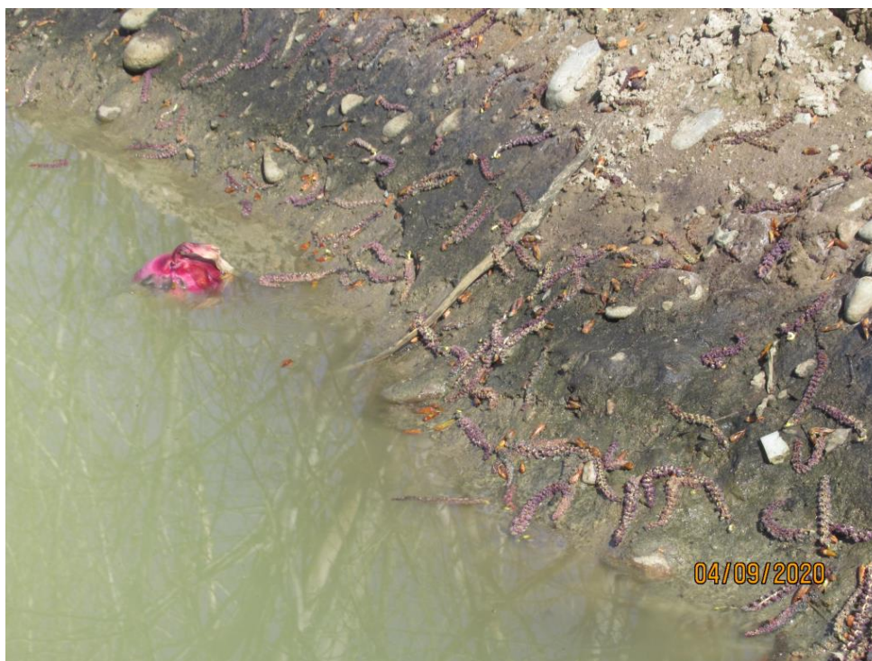
Photograph 44 :Close-up view of Swale #3, northeast end, note discoloration of soil, appears to be oil or petroleum based.
