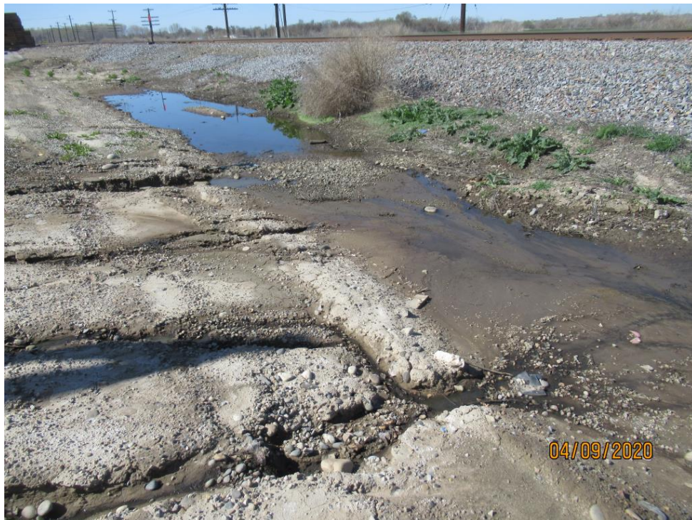
Photograph 76 :Rills and waste water from truck loading operations.
