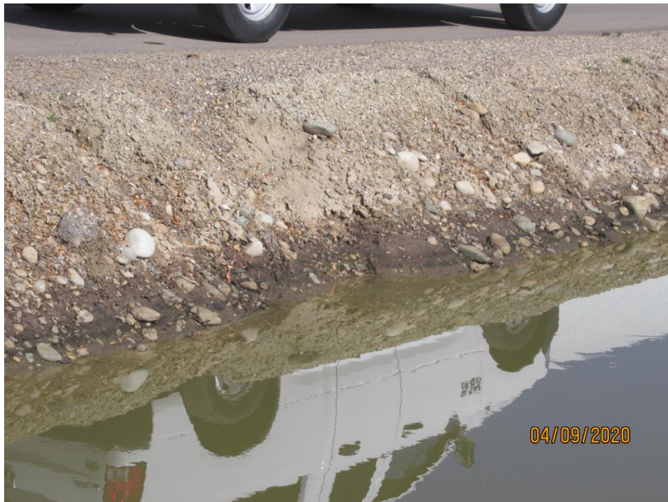
Photograph 30 :Rills on west bank of Swale #2 near south end of the swale.
