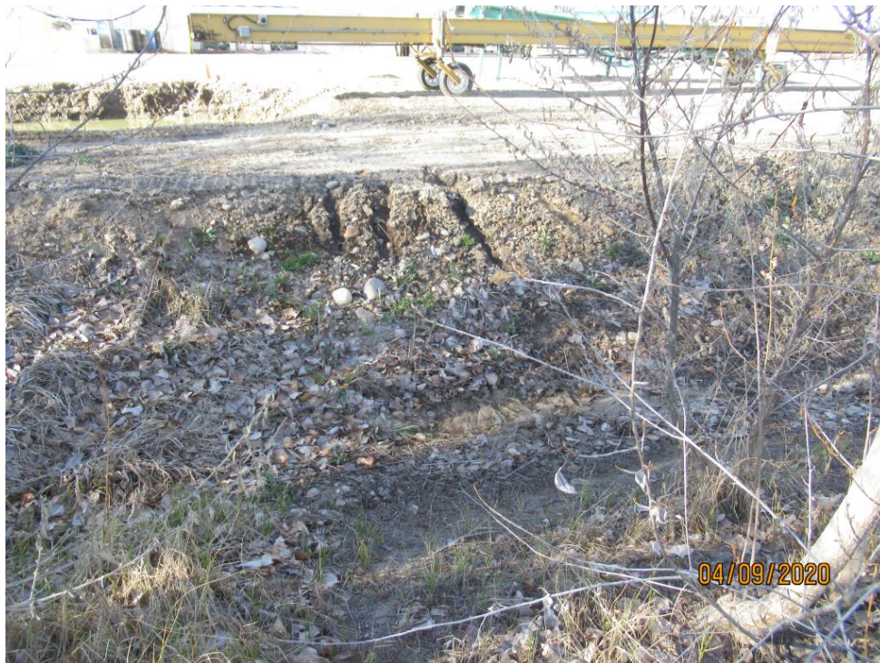
Photograph 12 :Rills on the north side of the facility, irrigation ditch is in the foreground, looking south.
