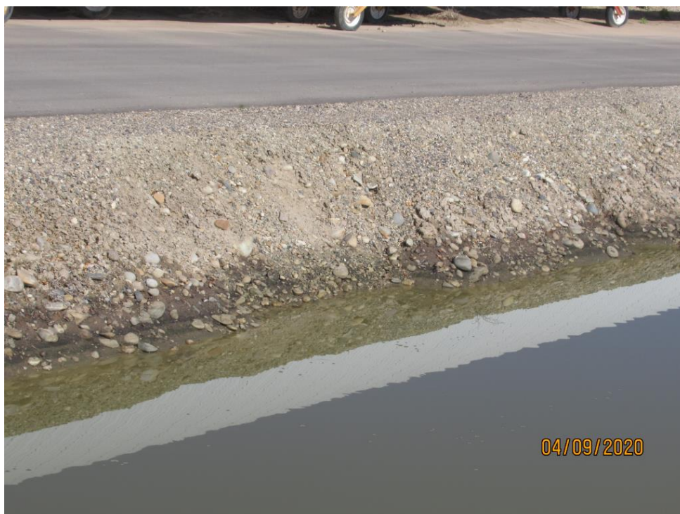
Photograph 32 :Close-up view of west bank rills, mid-way, Swale #2.
