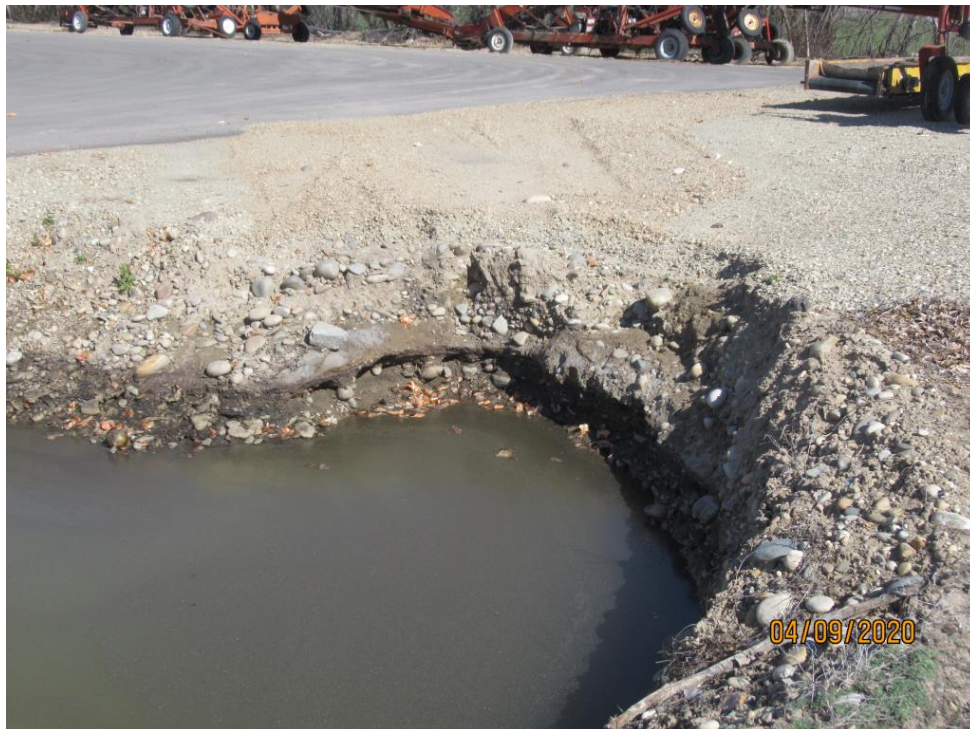
Photograph 36 :Close-up view of erosion area, Swale #2, north end.
