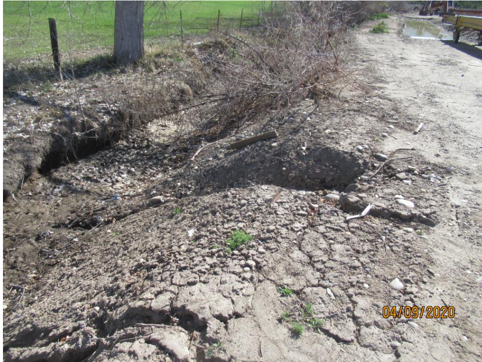
Photograph 61 :Large rill on facility property into north side irrigation ditch, looking east.
