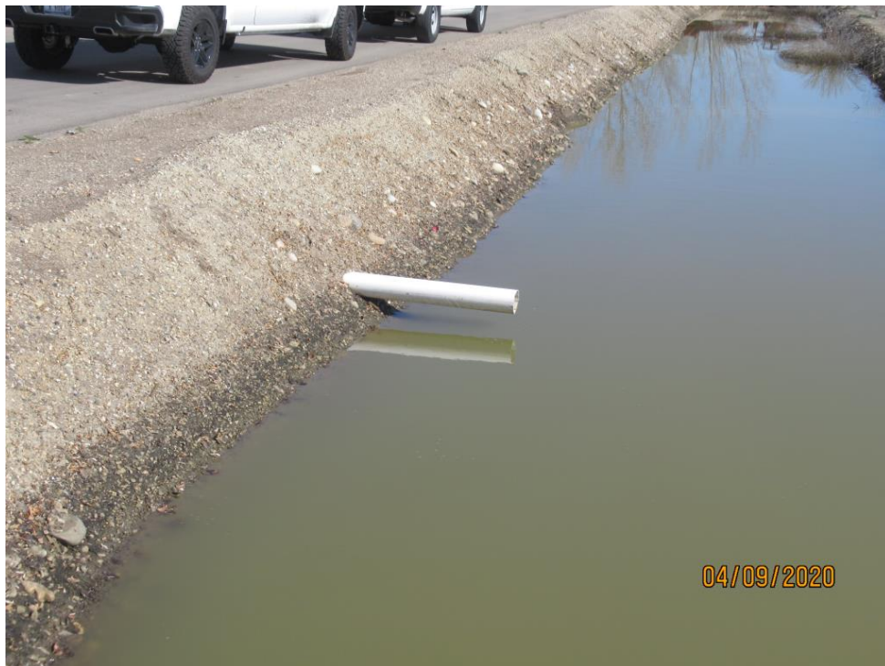
Photograph 28 :Stormwater outfall to Swale #2, looking north.
