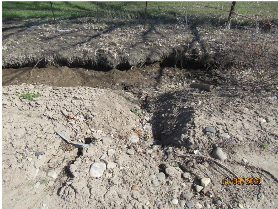
Photograph 62 :Large rill on facility property into north side irrigation ditch, looking north.
