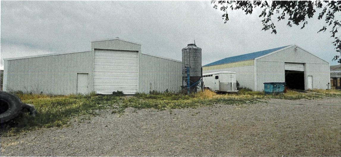
Barn to be Converted (left structure with garage door closed)
